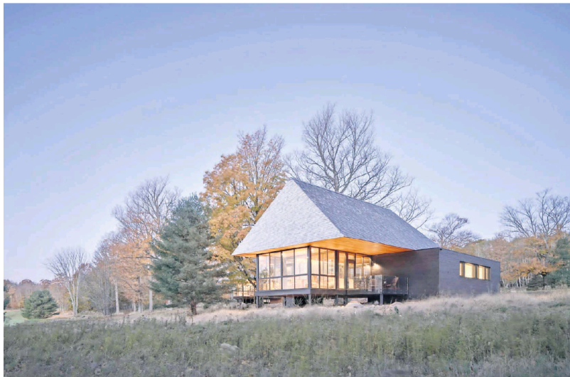
The Bigwin Island cabins designed by Halifax firm MacKay-Lyons Sweetapple are built around three main components: a rectangular great room, a “bed box” and a hipped roof with large overhangs. The blocks can be combined into many permutations. PHOTOS BY DOUBLESAPCE
